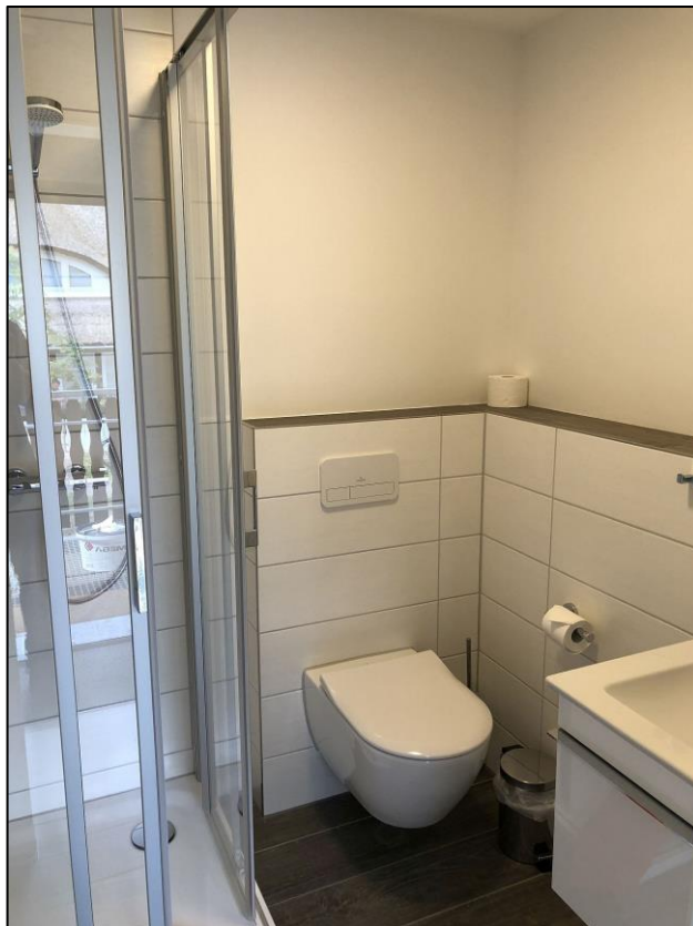
Blick in das neue Bad
